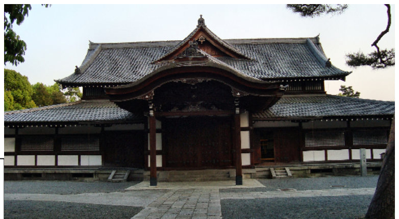
The Butokuden – The Hall of The Classical Martial Arts of Japan
